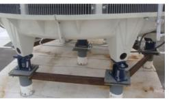
the center of each basin leg for this purpose. The factory can provide you with the basic mounting dimensions to aid in platform construction.
