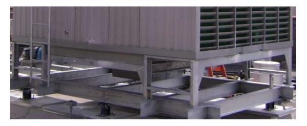
3.2 VIBRATION ISOLATION: Although vibration Isolators are not required, it is acceptable to use them as prescribed by local mechanical code. Consult the factory for specific on your model as necessary. If Isolators are employed, you would also need to use flexible connectors in the associated water lines.
