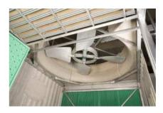
c. Inspect the Fan Blade making sure the retaining nut and u-bolts are tight. Spin the blade by hand making sure it is free of obstructions
