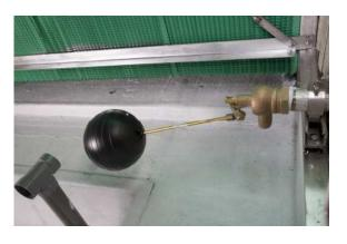
4.3 FRESH WATER MAKE-UP: The Fresh Water Make up is sized to replace evaporation and water bleed or blow-down. The factory provided float assembly is mounted with the necessary air-gap and no back flow prevention device is generally required. Any modification to this system done by the owner/operator needs to be done in accordance with the prevailing electrical codes and requirements.
