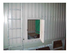
2.3 SERVICE ACCESS: RSS Series Cooling Towers are very reliable and need minimal maintenance. When selecting an installation location, be certain that you will have sufficient access in order to perform routine inspections and repairs as needed. Access doors and ladders should be positioned so that may be used in a safe and secure manner. If the tower is to be mounted above ground, refer to the prevailing mechanical code to ensure the safety of inspection and service personnel.
