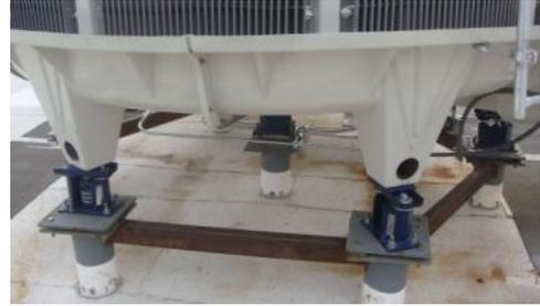
Towers that are installed on any raised platform must be firmly secured. There is a mounting hole in the center of each basin leg for this purpose. The factory can provide you with the basic mounting dimensions to aid in platform construction.
