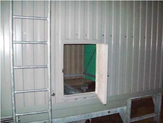
**2.3 SERVICE ACCESS:** RSS Series Cooling Towers are very reliable and need minimal maintenance. When selecting an installation location, be certain that you will have sufficient access in order to perform routine inspections and repairs as needed. Access doors and ladders should be positioned so that they may be used in a safe and secure manner. If the tower is to be mounted above ground, refer to the prevailing mechanical code to ensure the safety of inspection and service personnel.
