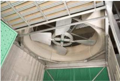
c. Inspect the Fan Blade making sure the retaining nut and u-bolts are tight. Spin the blade by hand making sure it is free of obstructions
