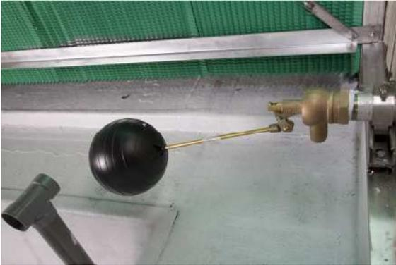
**4.3 FRESH WATER MAKE-UP:** The Fresh Water Make up is sized to replace evaporation and water bleed or blow-down. The factory provided float assembly is mounted with the necessary air-gap and no back flow prevention device is generally required. Any modification to this system done by the owner/operator needs to be done in accordance with the prevailing electrical codes and requirements.
